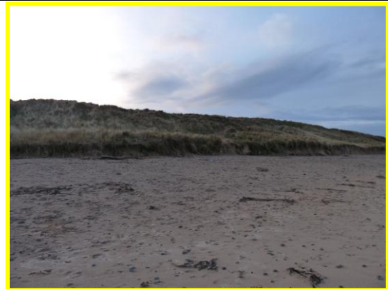
E52/8 – Consistent toe erosion throughout unit but limited in its extent upslope. December 2013 (Locally Active)
