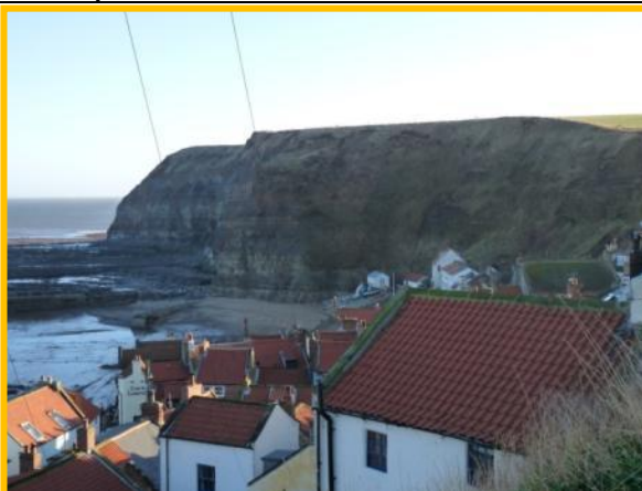
MU4/2 – Cliff behind Staithes harbour. No notable change post December 2013 surge except lack of talus accumulation. (Partly Active)
