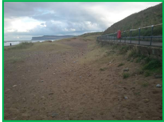
E52/7 Sand dunes and walls to toe of vegetated slope (Dormant) Photo October 2012
