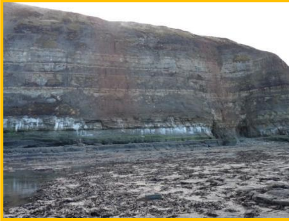
MU4/3 – undefended cliff east of Staithes Harbour. Note red-brown ‘streaking’ on cliffs from failures in till.
