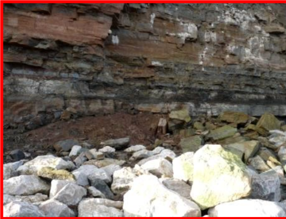
MU4/1a - Close up photo of talus accumulation behind rock armour after the December 2013 surge. (Totally Active)
