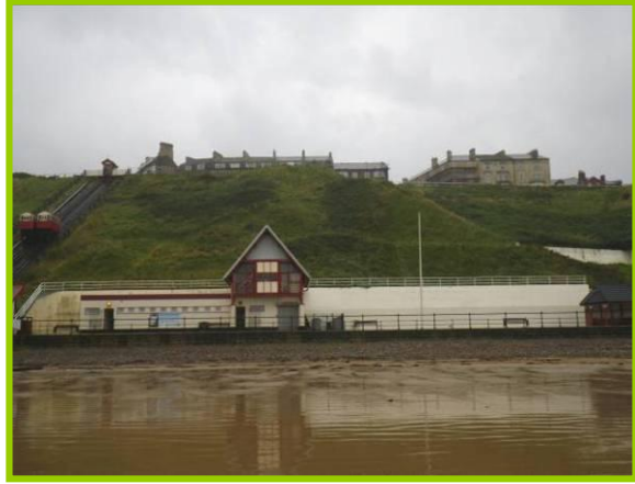
E52/3a the stabilised slopes close to the Cliff Lift (Inactive) September 2013
