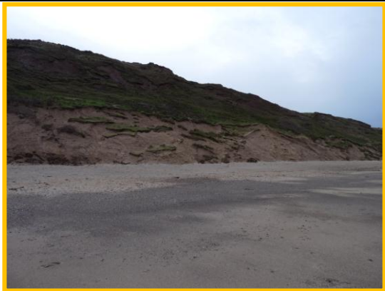
E52/4 – Significant toe erosion in sandy material and turf detachments above. Northern part of unit. December 2013. (Partly Active).
