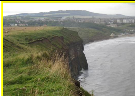
E53/3 and E53/2 The rock part of the cliff is steep and exposed. The till part is much shallower and vegetated (Locally Active). September 2012
