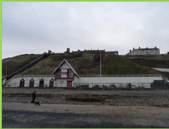
MU52/3a – Views from North (top left) to south (bottom right). Slope is defended but minor shallow instability noticed at several places in units. Repairs ongoing adjacent to cliff lift. Note accumulation of large volumes of coarse material (in piles, bottom right photo). December 2013. (Inactive).
